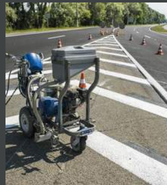
Signage & Pavement Marking
